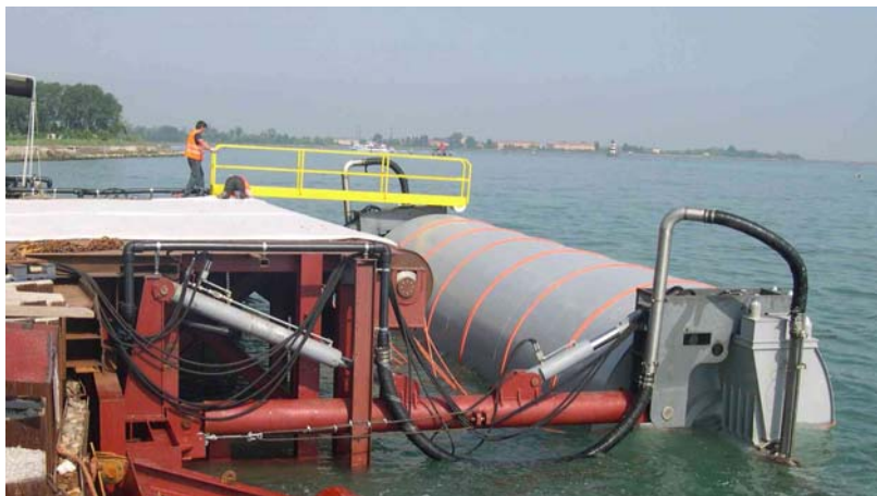
Figure 7: The drum before the BFM is wound
