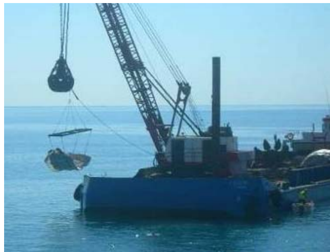
Figure 15: Special BFM laying down phases
