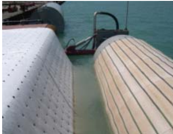
Figure 4: Mattresses being rolled onto the drum
