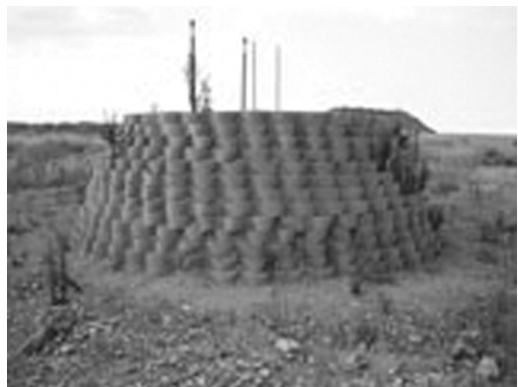
Figure 1. Test embankment in 700 days since construction.
