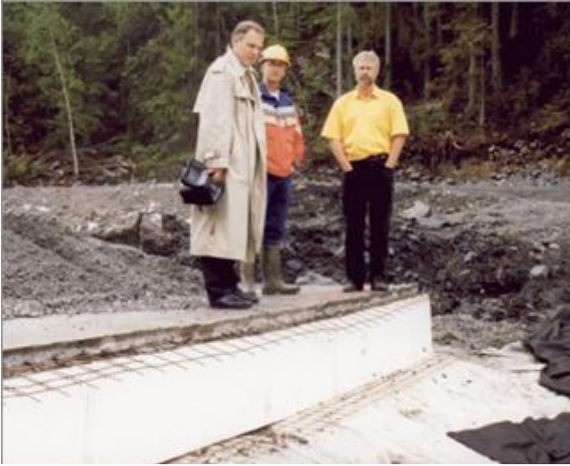
Figure 2. Example of concrete layer with light reinforcement over EPS blocks, above which the roadbase courses are subsequently followed by asphalt layers
