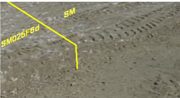
Figure 8. Compaction stage using a motor-scraper
