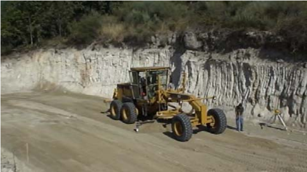
Figure 3. Preparation of an adequate foundation
