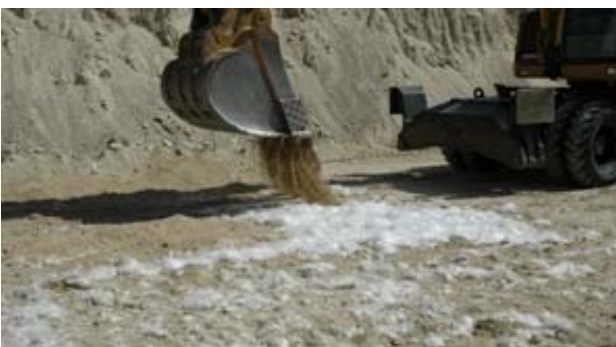
Figure 5. Thin soil and fibre layers placed alternately
