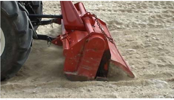
Figure 6. Mechanical mixing by means of a recycler type mixer
