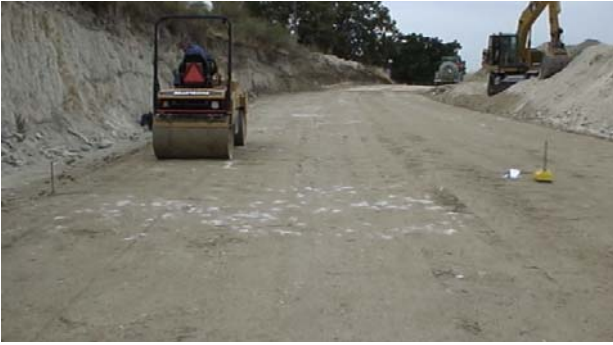
Figure 9. Compaction stage using a vibrating roller
