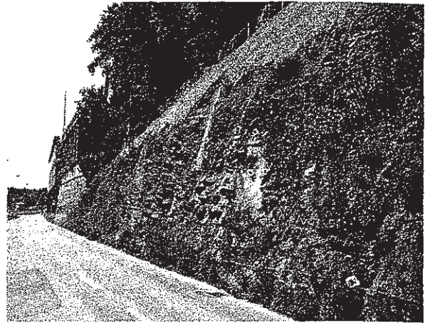
Figure 18. Protected slope (rocky section).
