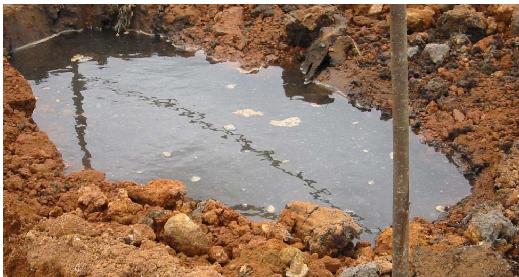
Figure 2. Water oozed out (and collected in a 1m long pit) when high pore pressure was created in peat with heavy tamping.
