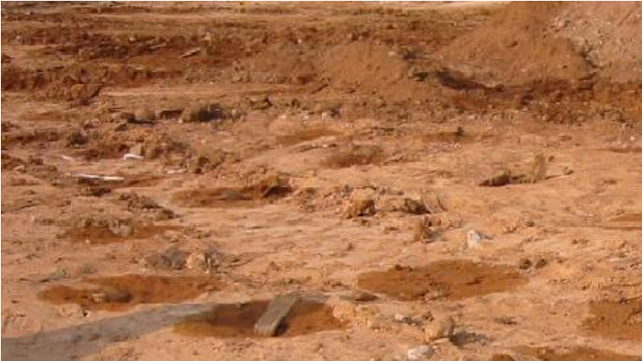
Figure 7. Vertical drains nearby tamping location (within 5m radius) conducting water
