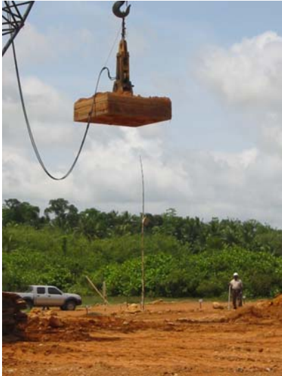
Figure 1. 80 Tonne crane lifting 15 tonne steel pounder to be released hydraulically
