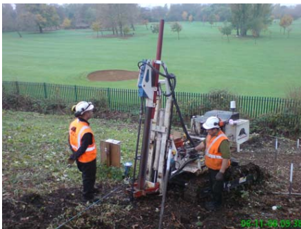
Figure 9 Installation of anodes and cathodes
