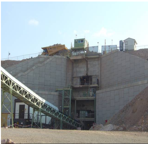
Figure 6. Retaining walls for the primary crusher of Kisladag gold mine Usak, Turkey (22.5m)
