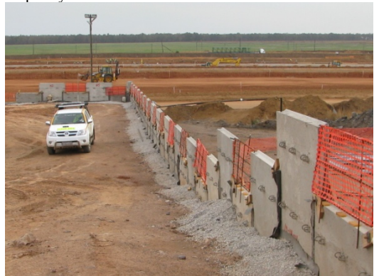
Figure 3. Drainage behind the concrete panels
