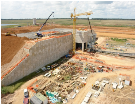
Figure 1. MSEW Macforce retaining wall
