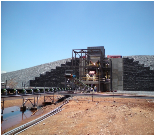
Figure 4. Combination of Macforce and Terramesh Aflease Gold mine South Africa
