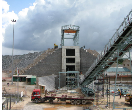
Figure 2. Terramesh gabion MSEW with geosynthetic soil reinforcement (Iduapriem Ghana)
