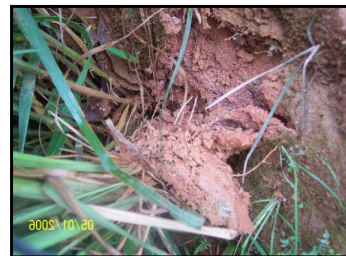
Photo 3 Roots penetration into the slope anchors the system.
