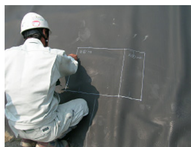
Fig.2 Marking of geomembranes
