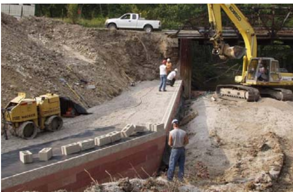
Figure 7. Construction of GRS Abutment
