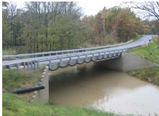
Figure 8. Completed Bowman Road Bridge
