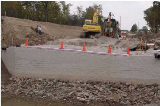
Figure 4. Face View of GRS Abutments to Show Bridge Super Elevation
