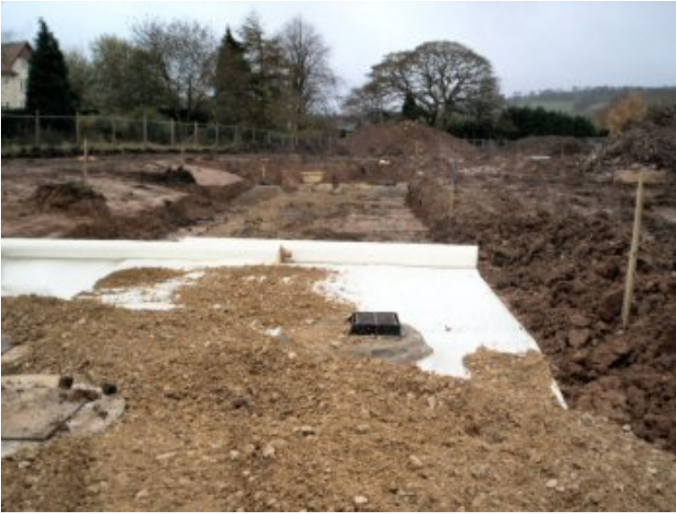
Figure 8. Geotextile installation under road
