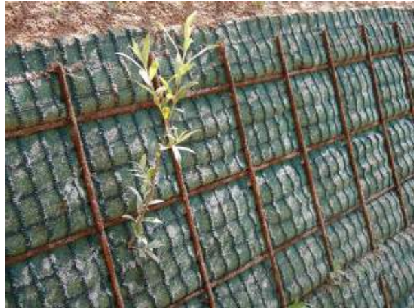
Figure 13. The new geogrid on the face of a vegetated reinforced slope
