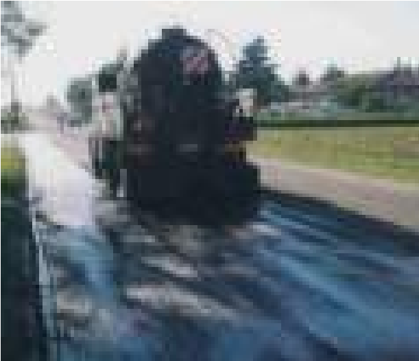
Figure 4. Spraying of the tack coat through a tank truck with spraying bar
