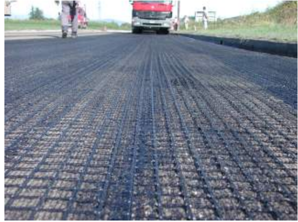
Figure 3. Two workers can lay down a whole roll of geogrids, 100 m long, in few minutes
