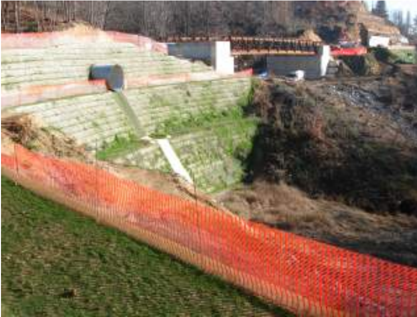
Figure 16. Road embankment and wing walls, showing the excellent quality of the vegetation and naturalization.
