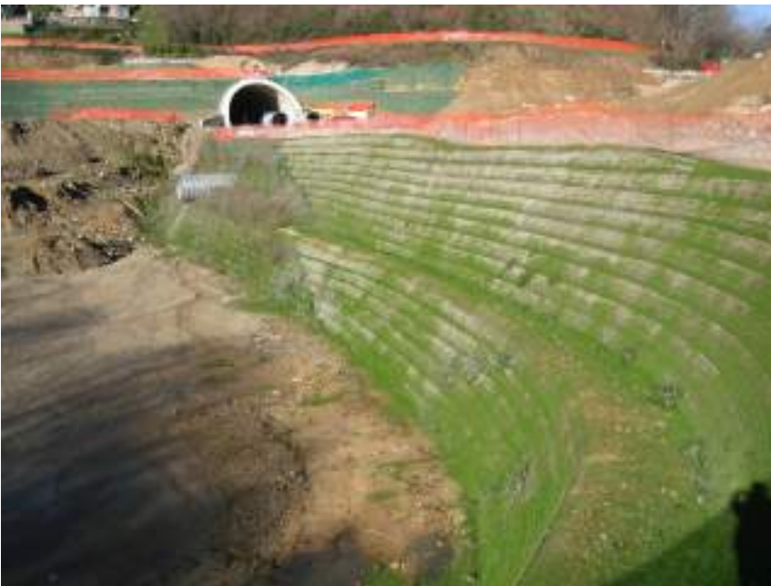
Figure 15. Reinforced soil structures at tunnel exit in Cossato, showing the growing vegetation
