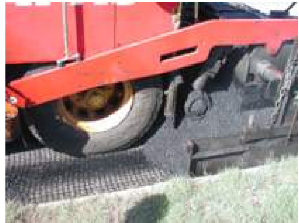
Figure 7. Laying the asphalt by a finisher
