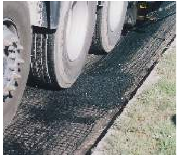
Figure 5. A small quantity of asphalt allows to keep the geogrid roll in the right position
