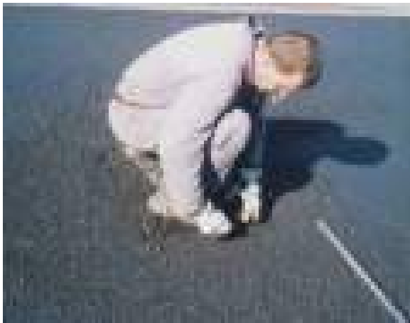
Figure 6. Manual cut of the geogrid around hitches or traps
