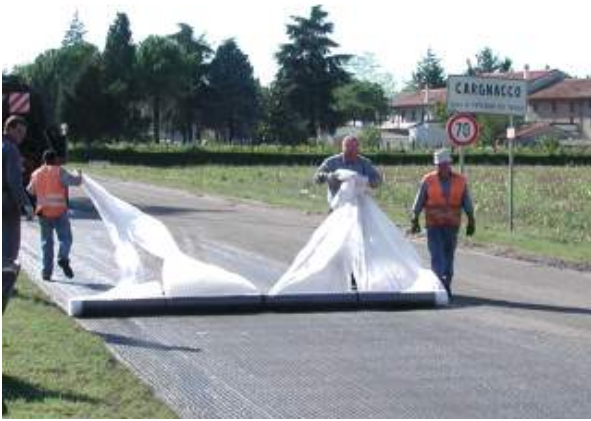
Figure 2. By pulling the Polyethylene sheet, the geogrid unrolls uniformly on the support layer, without creating folds or waves
