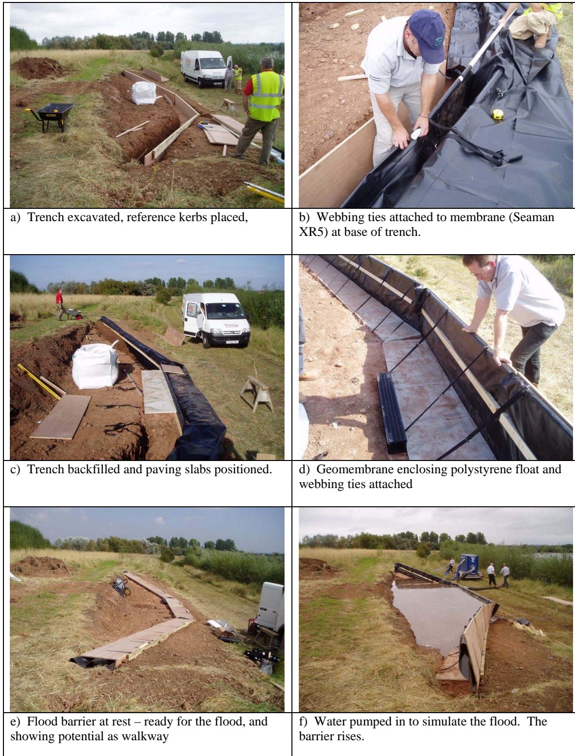
Figure 3. Stages of construction and operation of the barrier during pilot trials.
