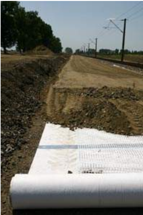
Figure 10. Installation of FPL on RDG and geogrid
