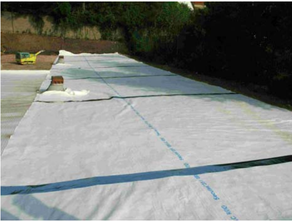
Figure 1. Mechanically bonded geotextile with aluminium reflector strips (RDG)
