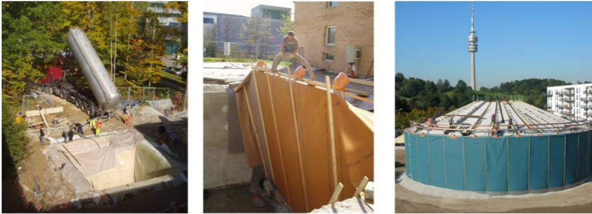
Figure 5. Bulk insulation material in membrane-formwork with diffusible liner (source, ITW: left and middle, Solites: right, SNAB, München-Ackermannbogen)
