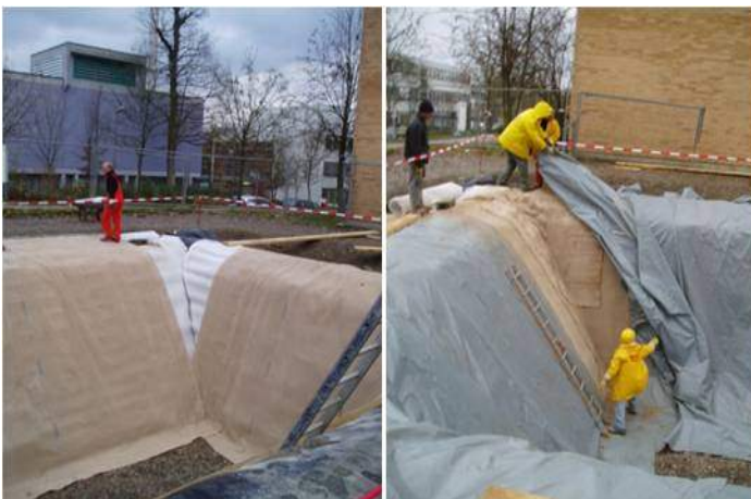
Figure 9. Installation of the GCL in outdoor laboratory
