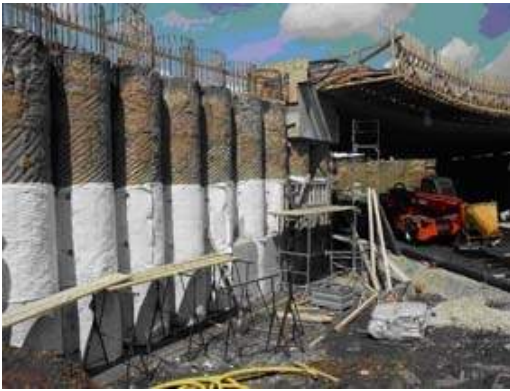
Figure 1. A geodrain being installed on the B529 Herford Bypass, Germany
