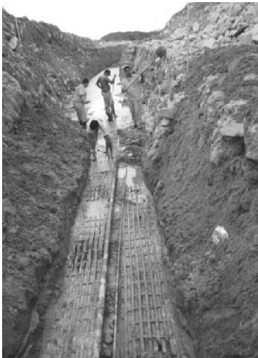
(b) Excavation to locate geogrid failure.
