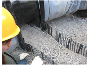
Figure 7. Installation of geogrid
