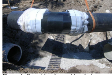
Figure 6. Geogrid and a steel bend pipe
