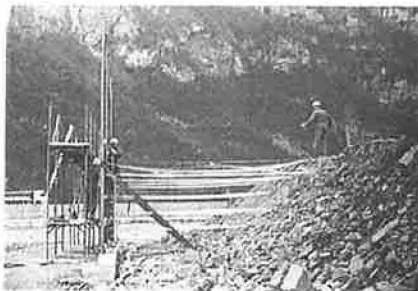
figure 5: wires and control panel for reinforcements displacements mesures (Trento Wall)
