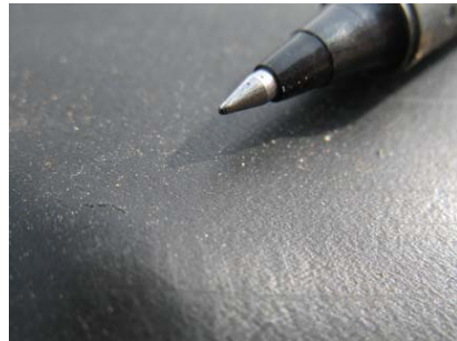
Figure 2 Small crack (circled) at subgrade stone protrusion
