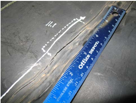
Figure 5 Stress cracks along extrusion weld
