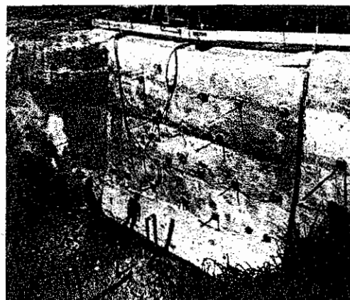
Fig. 1 First scientifically tested wall in the history of soil nailing 1976 (wall after failure)
