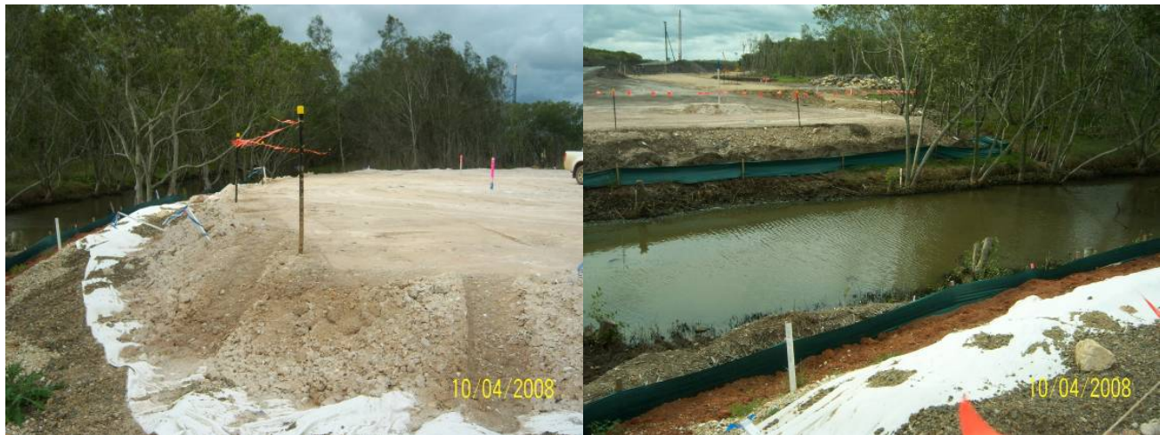
Figure 7. The fabric installed at BR25A and BR25B
