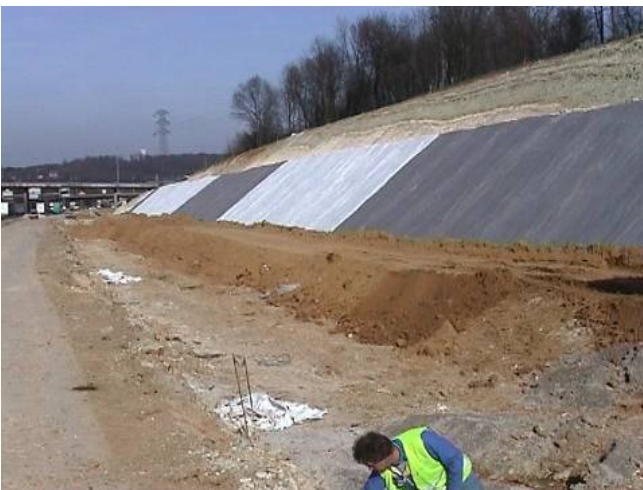
Figure 13. Filling, resurfacing and under-steeping the slope
