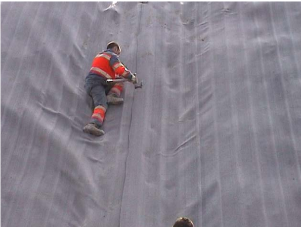
Figure 3. Drainage geocomposite fixation on the slope
