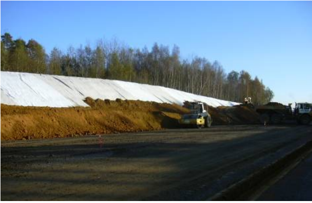
Figure 9. Filling, resurfacing and under-steeping the slope embankment
