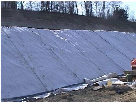
Figure 2. Application of the drainage geocomposite on the slope
