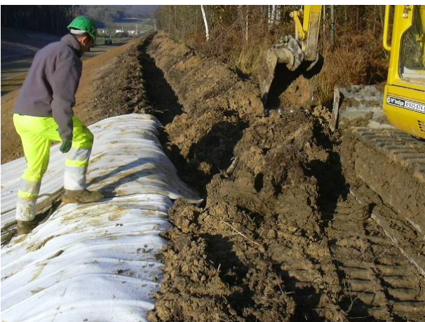
Figure 5. Mechanical fastening at the summit with anchoring
