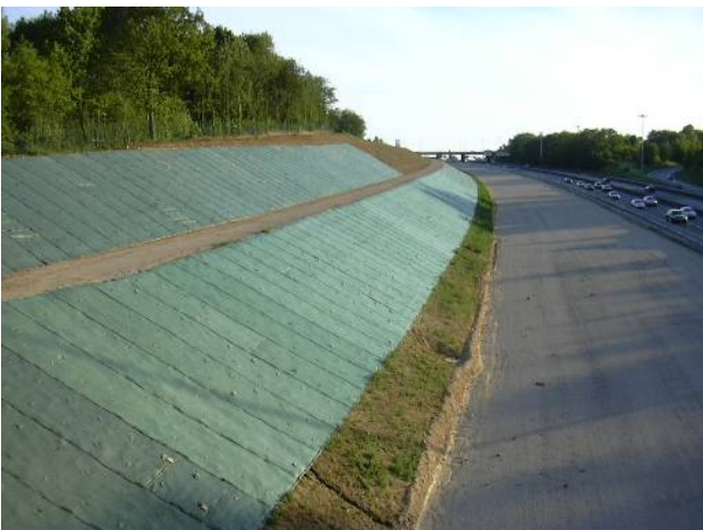
Figure 14. Completion of the cut slope
