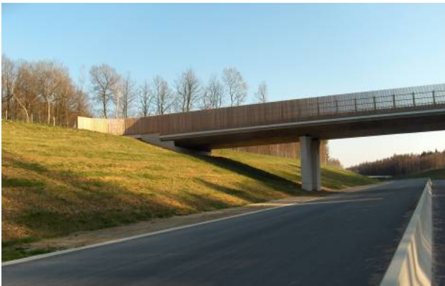
Figure 10. Completion of the cut slope
