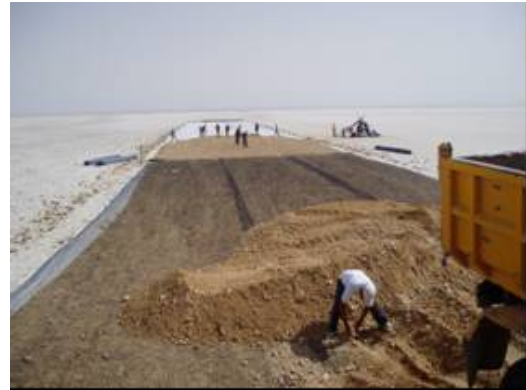
Figure 5. Laying the geogrid over the first lift of the embankment
