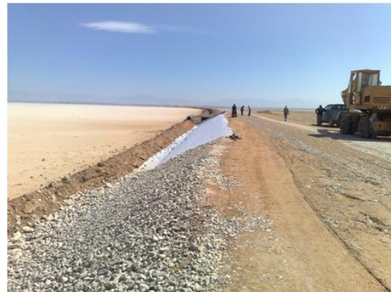
Figure 7. Protection of embankment slopes
