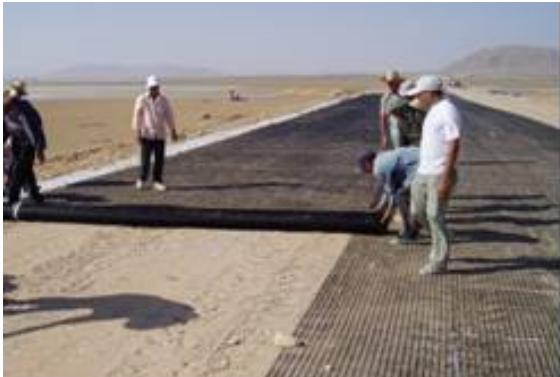
Figure 5. Laying the geogrid over the first lift of the embankment
