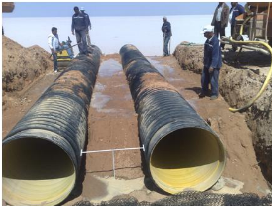
Figure 6. PEHD reinforced tubes installation
