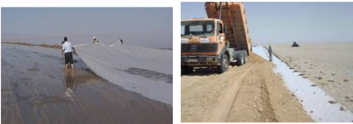
Figure 4. Laying directly over sabkha surface a nonwoven geotextile GT 1
