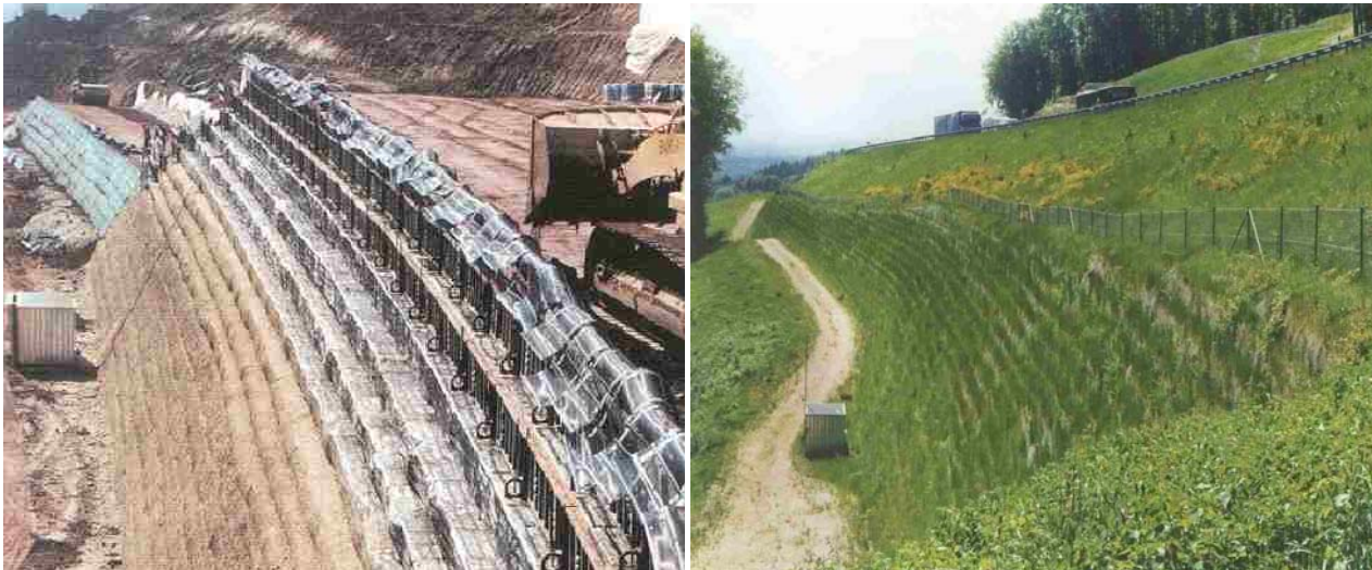
Figure 1. A9 during construction stage and after full vegetation
