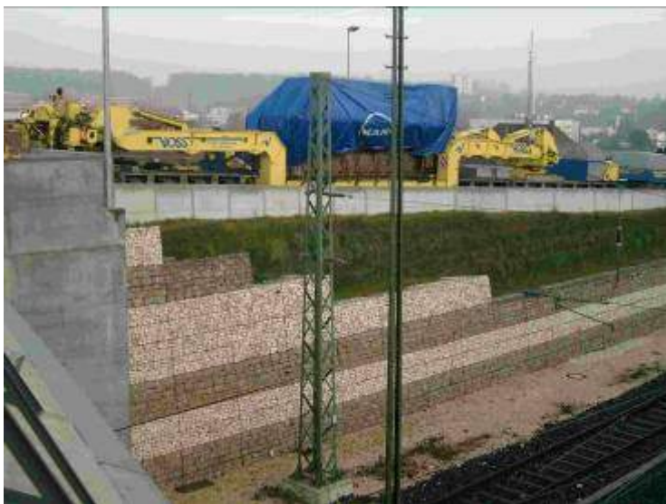
Figure 5. Condition during test-loading, measured settlement under the structure
