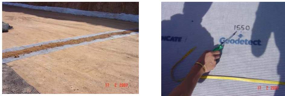
Figure 6. Placement of the 'intelligent' geosynthetic strip.
