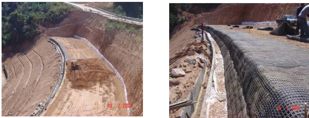
Figure 4. Slope failure at Maehongson and rehabilitation of the slope using geosynthetic reinforcement.
