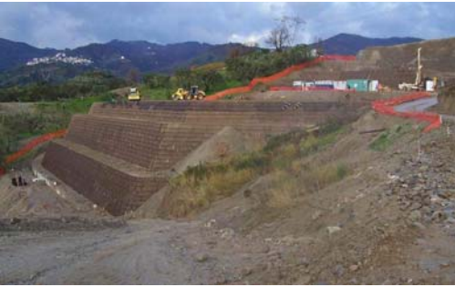
Figure 13. The 18m high earth reinforced slope is under construction.
