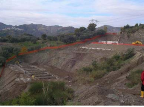
Figure 12. The construction of the foundation structure (lower left).
