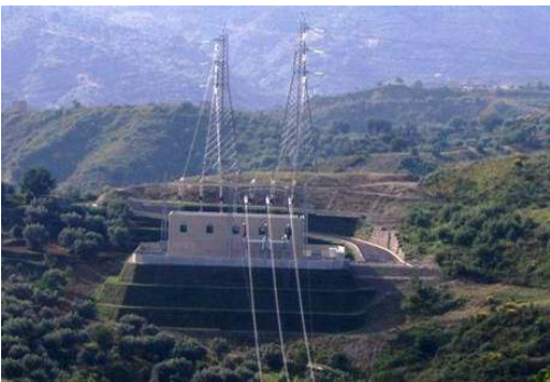
Figure 14. The transforming station after completing the works.
