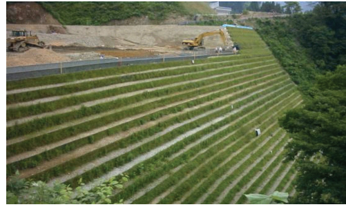
Figure 2. Overall view of TOGA wall.
