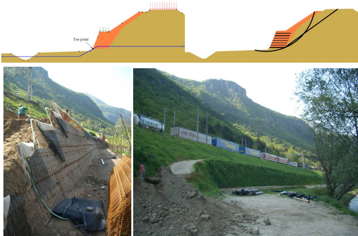
Fig. 11 - Stability analyses in condition of rapid draw-down and construction of the reinforced soil structure
