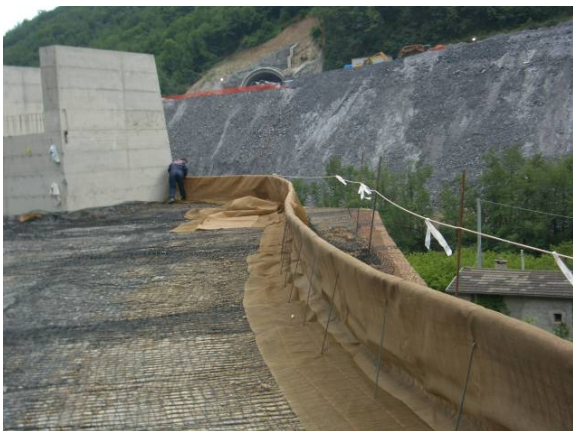
Fig. 6 – Photos taken during construction of the reinforced soil structures
