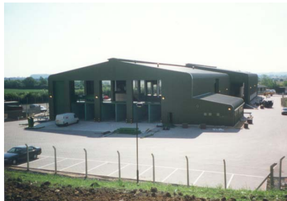
Figure 13. Waste transfer station in operation over Geocell Mattress foundations
