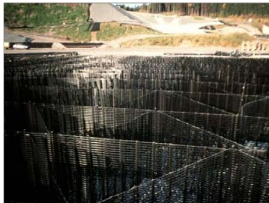
Figure 11. Geocell Mattress over tailing pond
