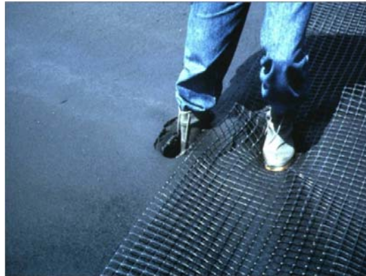
Figure 10. Biaxial geogrids provides working platform over very weak fill
