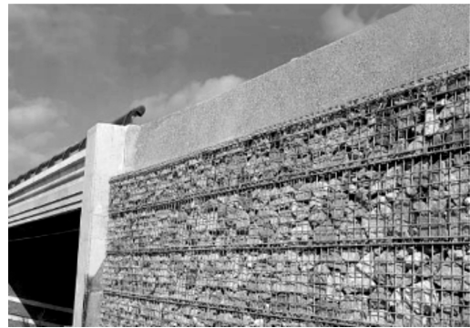
Figure 4. Wire-faced MSE Wall – 1H:4V Wall.
