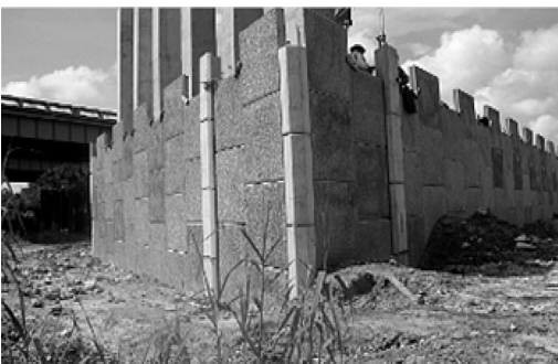
Figures 7 and 8. View of CMC rig and MSE Wall during construction.
