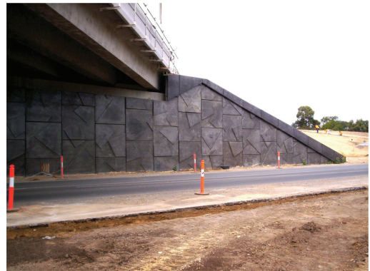
Figure 3. View of completed reinforced earth wall.
