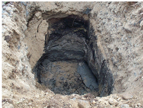
Figure 1. Typical test pit showing the condition of the uncontrolled fill.
