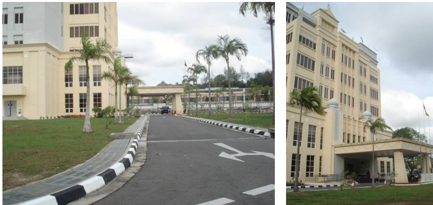
Figure 12. Situation at Bangunan City Hall after completed construction works
