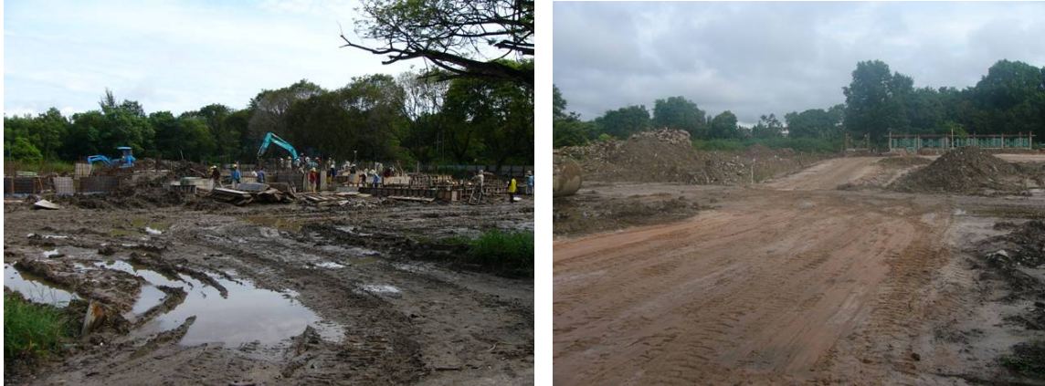
Figure 11. (left) Severe rutting in access road, (right) Improved access road condition with geocomposite
