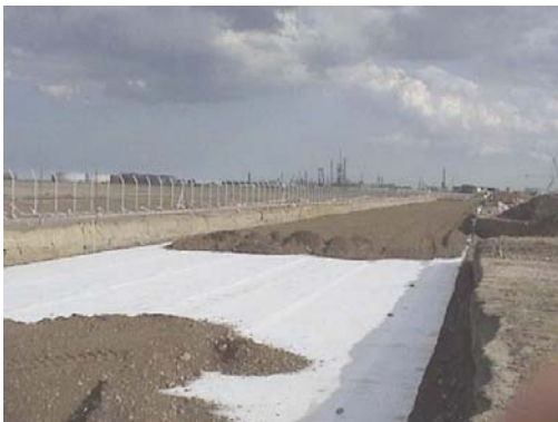
Figure 10. Installation of composite base course reinforcement
