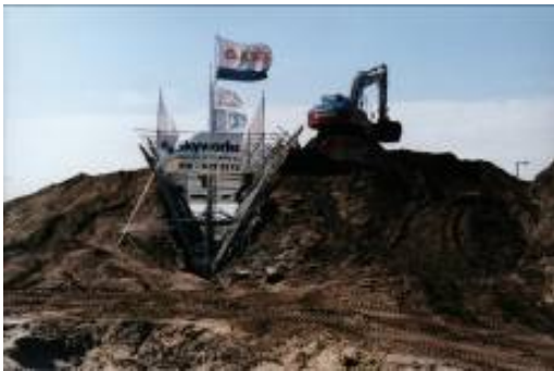
Figure 7. Scaffolding during construction
