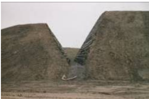
Figure 8. Cleft after finishing construction
