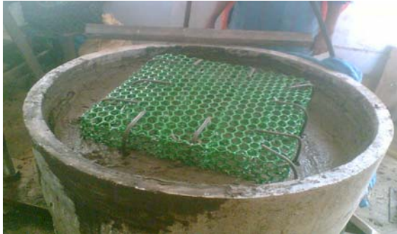
Figure 2. Cellular geogrid cage ready for pushing
