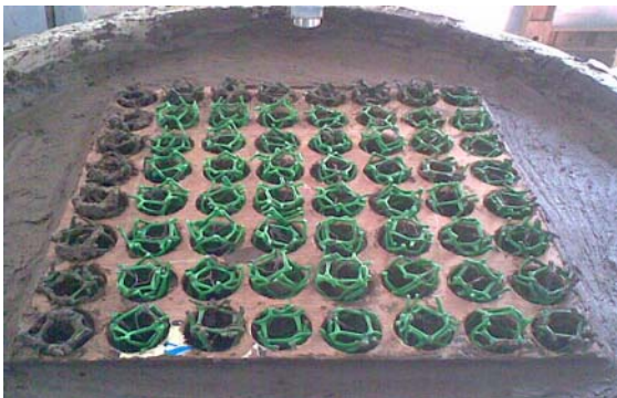
Figure 6. Installation of circular geogrid cage
