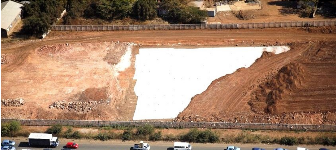
Figure 7: Aerial view of multi-layer geosynthetic reinforced embankment
