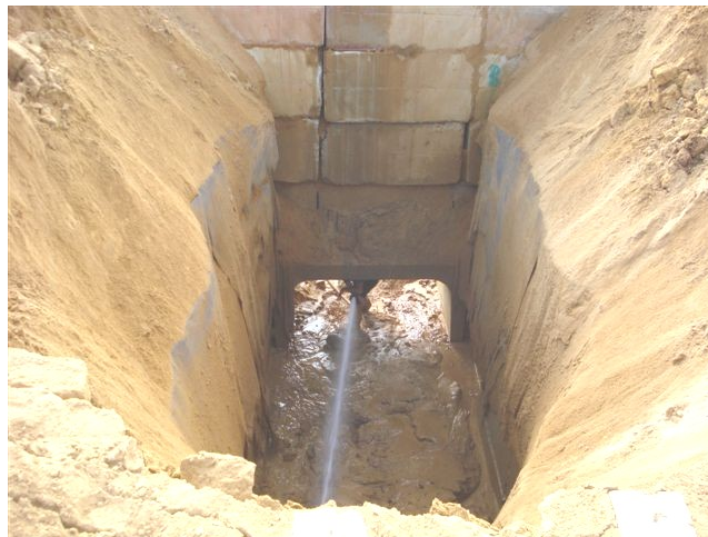
Figure 5: Undermined from below, the sides of the resultant trench were close to vertical
