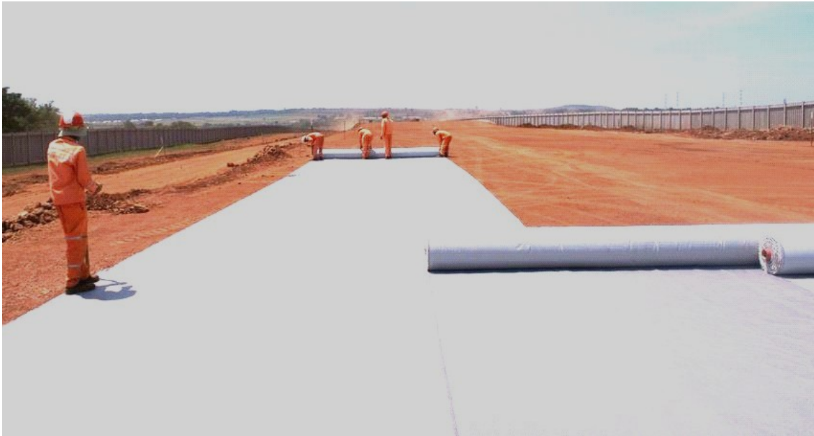
Figure 6: Laying composite geogrid
