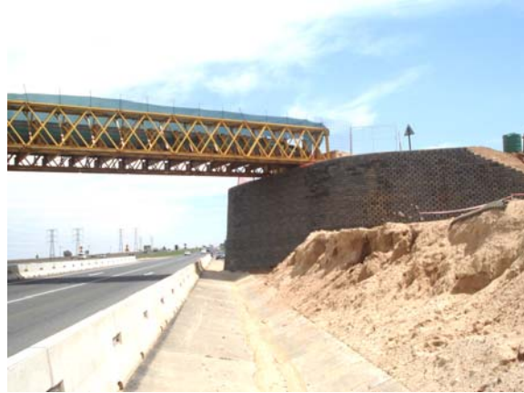
Figure 12: Abutment structure for a temporary bridge
