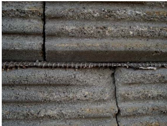
Figure 13: Trimmed and burnt back geosynthetic
