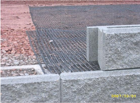
Figure 5. Showing Double Geogrid Connection
