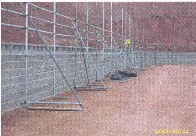
Figure 8. Wall Partly Built Showing Safety Barrier
