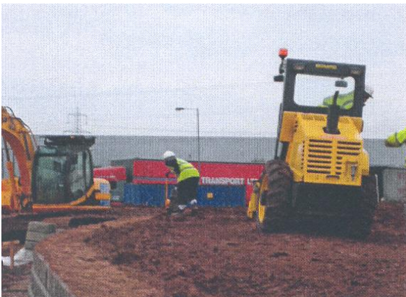
Figure 6. Laying and Compaction of Fill
