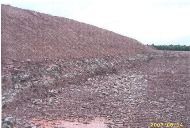
Figure 4. Showing Bulk Excavation
