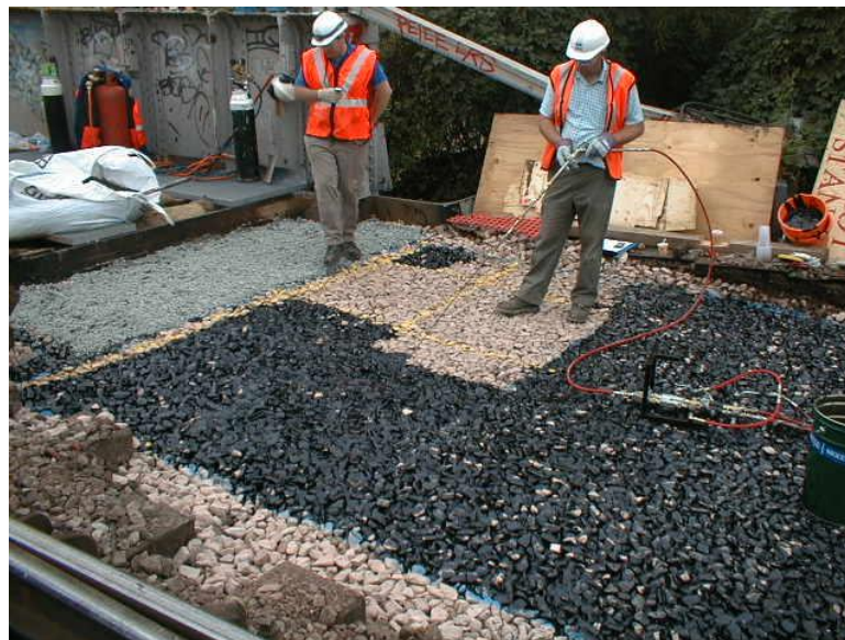
Figure 8. Formation of the lower polymer reinforcement at Tottenham South Junction, UK
