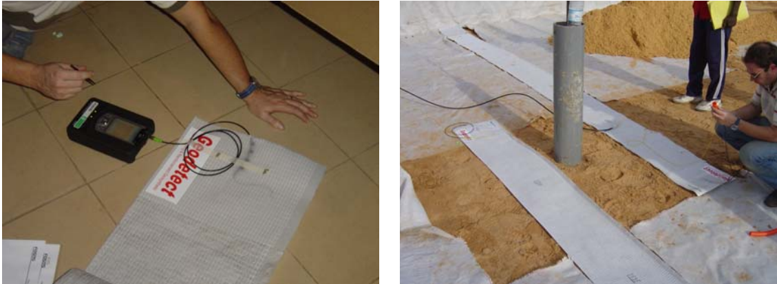
Figure 11: Strip control before installation and installation
