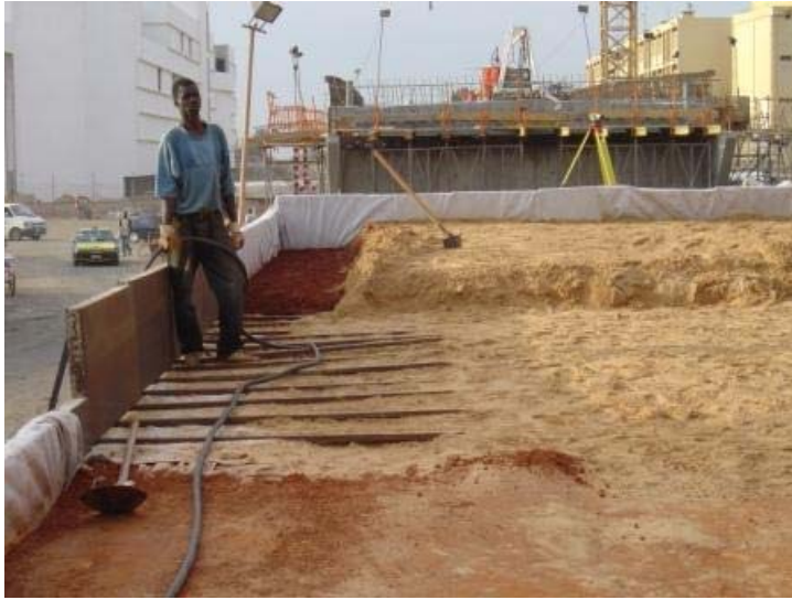
Figure 7: Temporary formwork, fill installation and compaction – « Malick SY »
