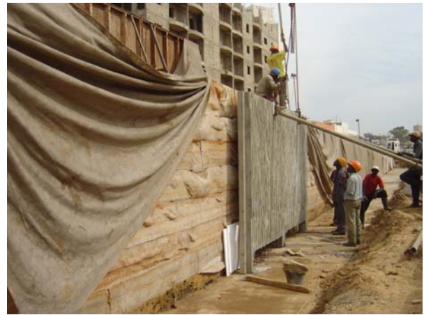
Figure 8: Fill elevation and prefabricated concrete panels installation – « Malick SY »
