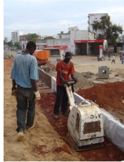
Figure 7: Temporary formwork, fill installation and compaction – « Malick SY »
