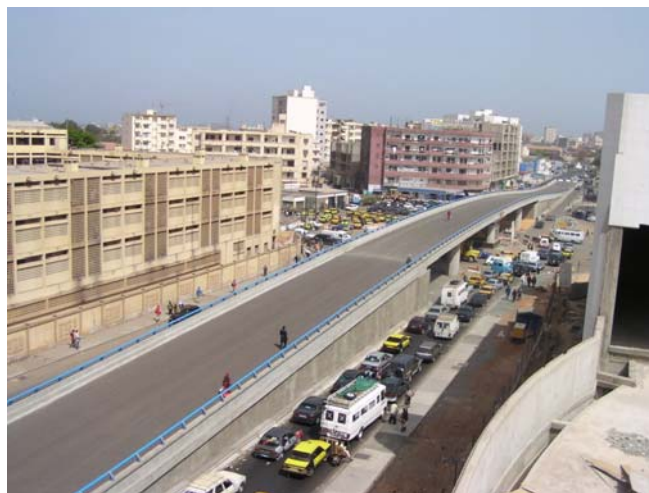
Figure 9: "Malick Sy" cross road completed.
