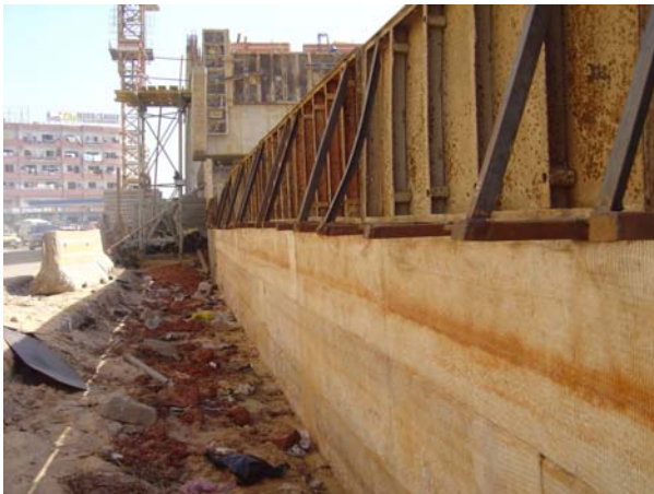
Figure 8: Fill elevation and prefabricated concrete panels installation – « Malick SY »
