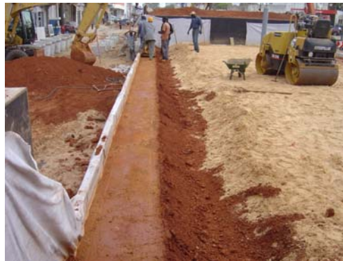
Figure 3: Dune sand peripheral confinement with laterite
