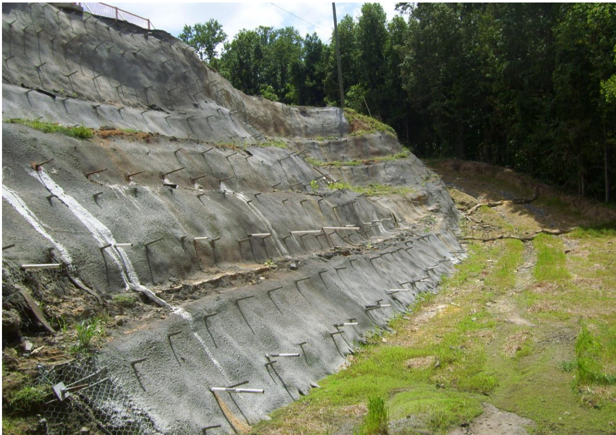
Figure 6: Temporary Shoring during Phase I
