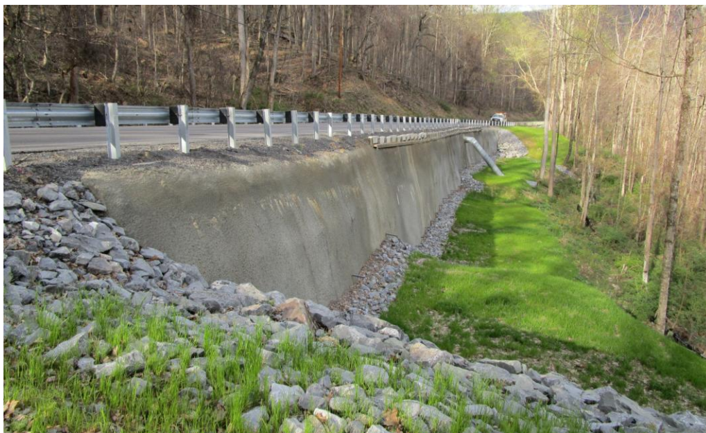
Figure 4: Soil Nail Wall Repair
