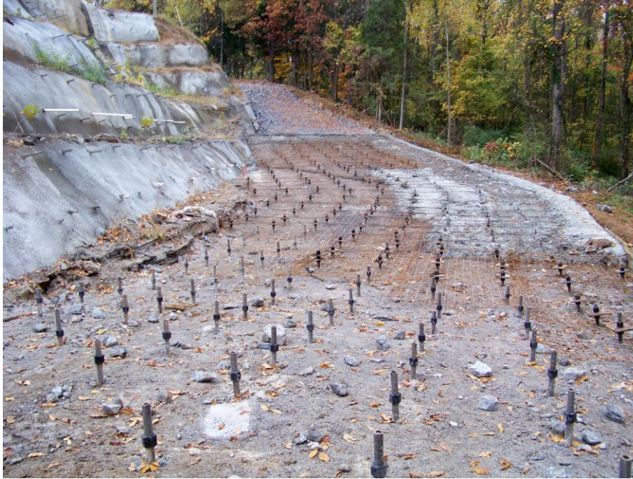
Figure 7: Micropile foundation during Phase 1
