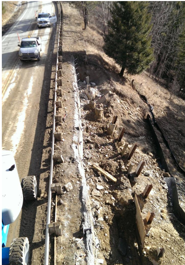
Figure 11: Existing Piling during Construction
