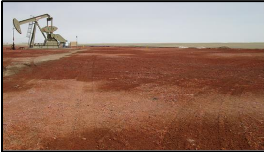
Figure 9. Well pad constructed with GTXw stabilization.
