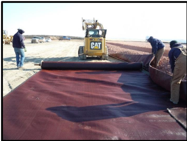
Figure 5. Geosynthetic material installed and overlapped 600 mm (24 in).
