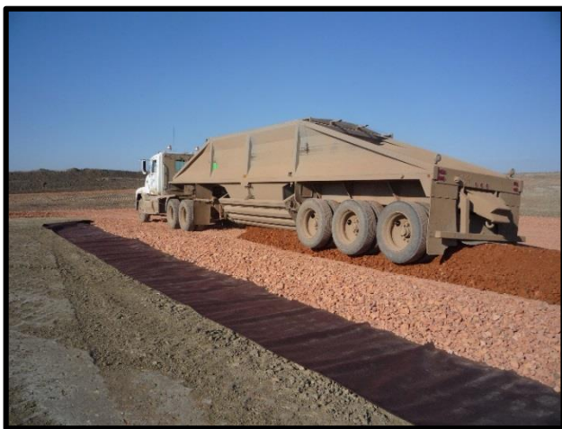
Figure 6. Aggregate placed onto the geosynthetic.
