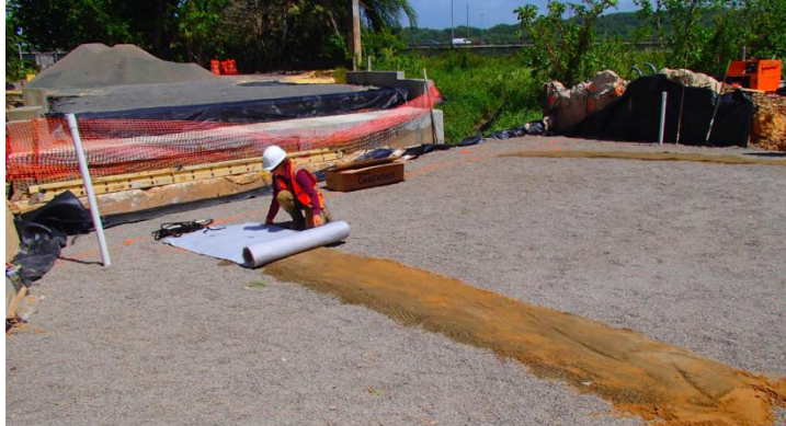
Figure 9: Geodetect® installation over layer of sand
