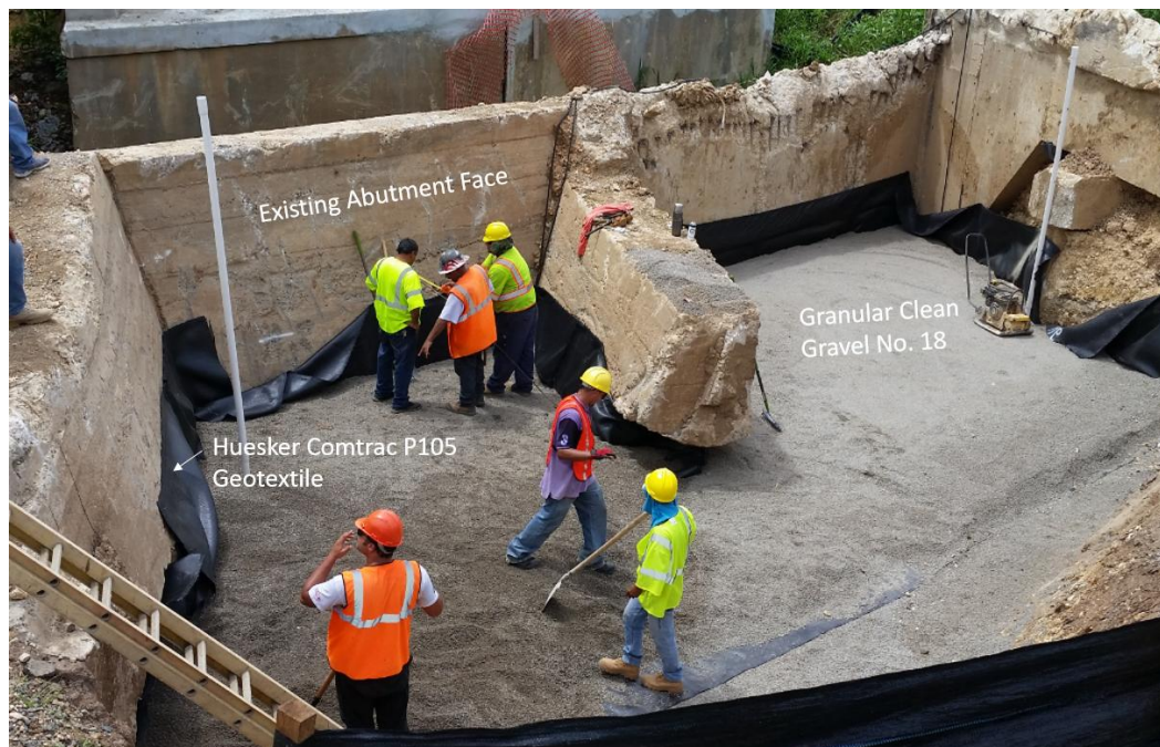
Figure 3: Construction of GRS abutment utilizing existing abutment face
