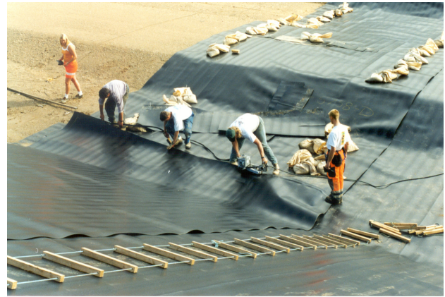
Figure 4. Illustrates the as-built condition regarding the GM part of the works.
