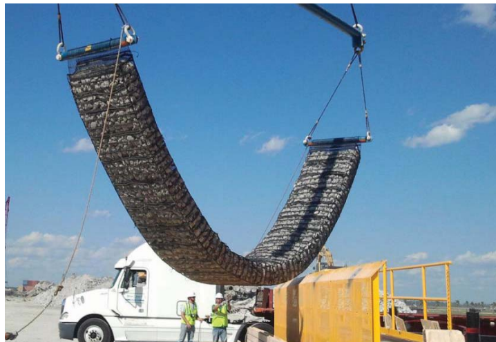
Fig. 25: Marine Mattress being hoisted from the filling frame (Fiske, 2015)
