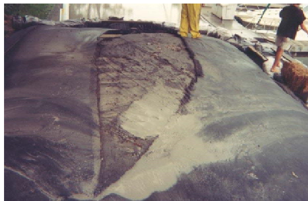
Fig. 24: Controlled failure of geotextile tube (Gaffney, 2013).
