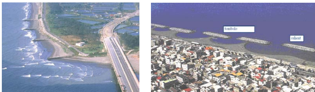
Fig. 18: Groins and offshore breakwaters coastline protection cases in Taiwan (Hsu, 2008).
