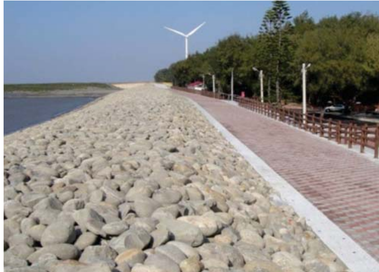
Fig. 6: Example of a revetment.
