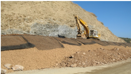
Figure 4 : Final aspect of stability toe embankment
