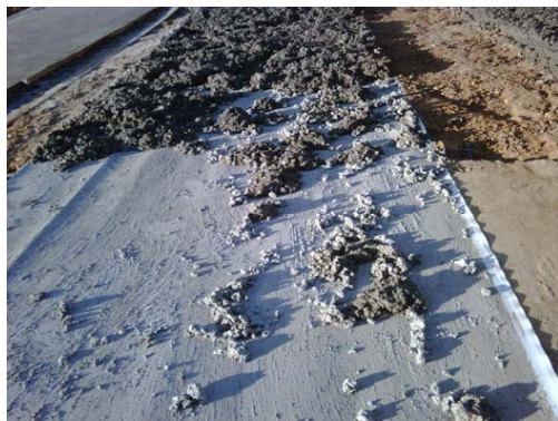
Figure 7. Detail of the smooth geomembrane surface after concrete placement.
