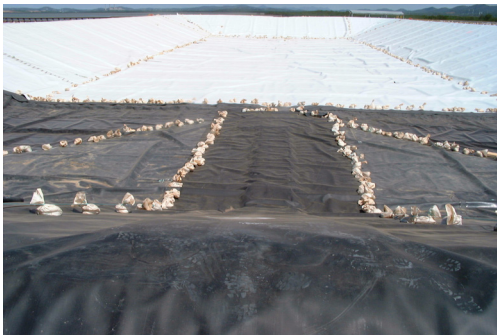
Figure 2. Construction of geotank base liner.
