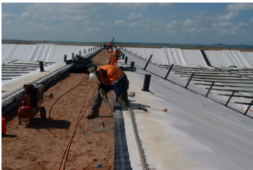
Figure 3. Construction of geotank cover system.
